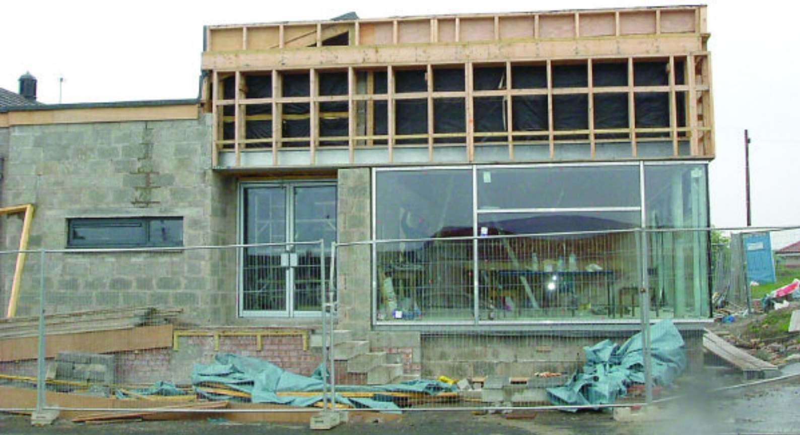
Under construction at Loganlea
