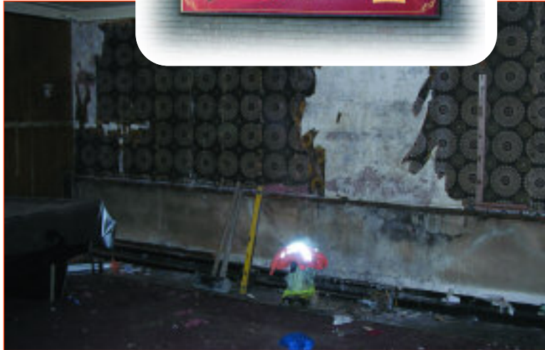
The work begins.
